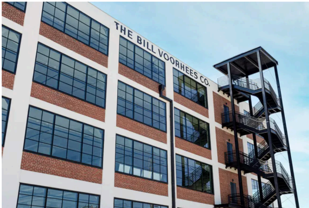
The historic Voorhees building in the Paseo South Gulch development. Derek Lee / Provided By SomeraRoad
