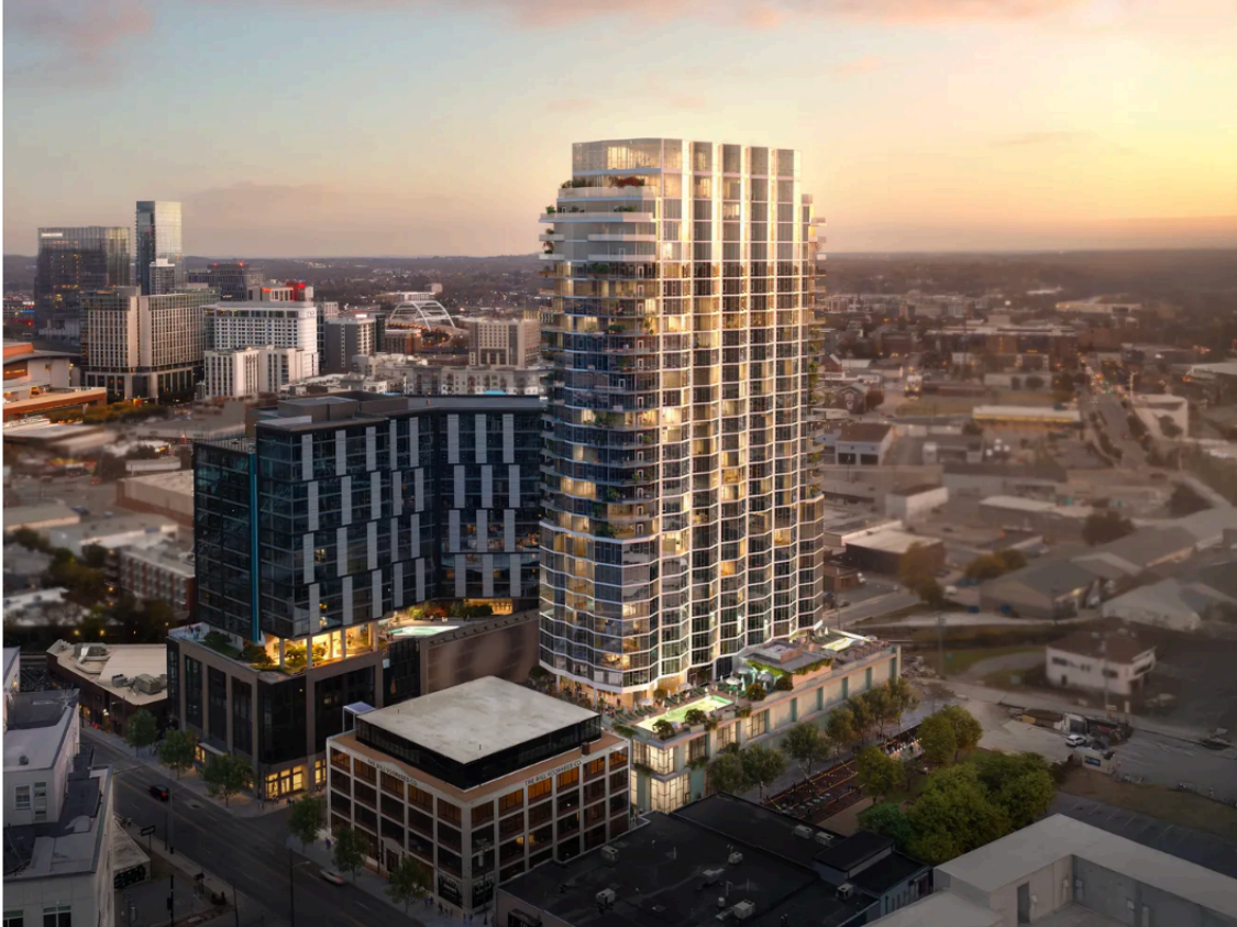
Pendry Nashville Hotel and Residences reveals details behind new real estate development, led by SomeraRoad in Paseo South Gulch. Provided By SomeraRoad
