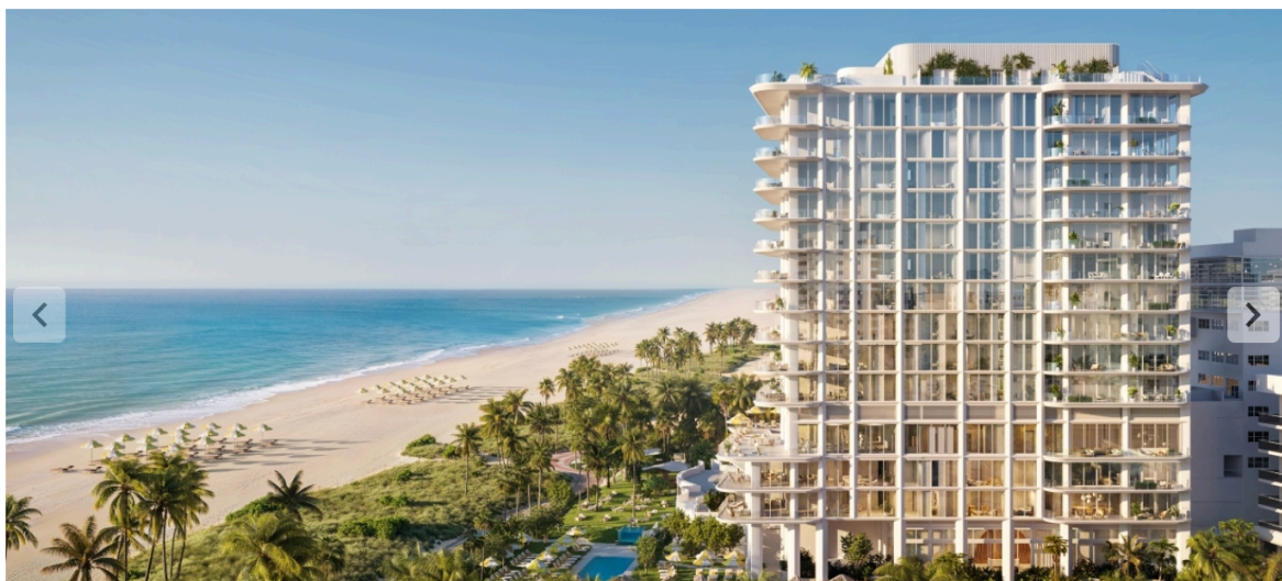
The Ritz-Carlton Residences, South Beach, in Miami Beach is integrated into the broader Ritz-Carlton and Sagamore hotel site. All renderings courtesy of The Boundary
