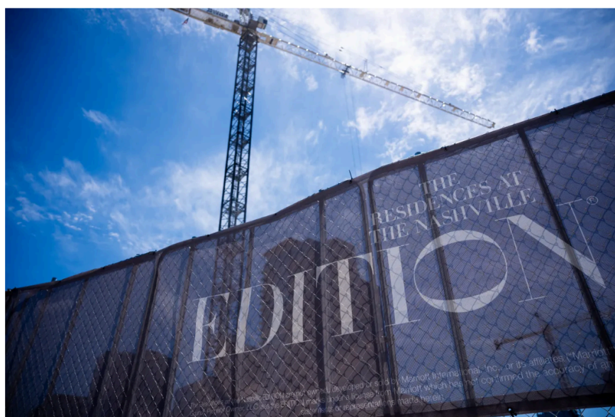
Construction continues at the site of a new hotel, Edition in Nashville on Friday, May 8, 2026. NICOLE HESTER / THE TENNESSEAN
